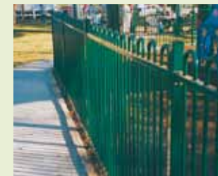
▼ The same fence re-coated in Plascoat PPA 571 after 6 years.
